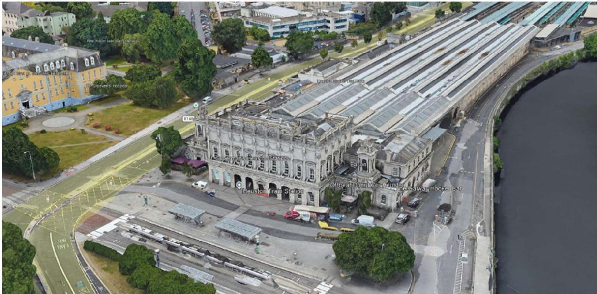
Figure 10 - Aerial View of Heuston Station
