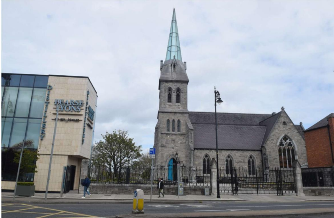
Figure 12 - Pearse Lyons Whiskey Distillery, Former St. James's Church of Ireland
